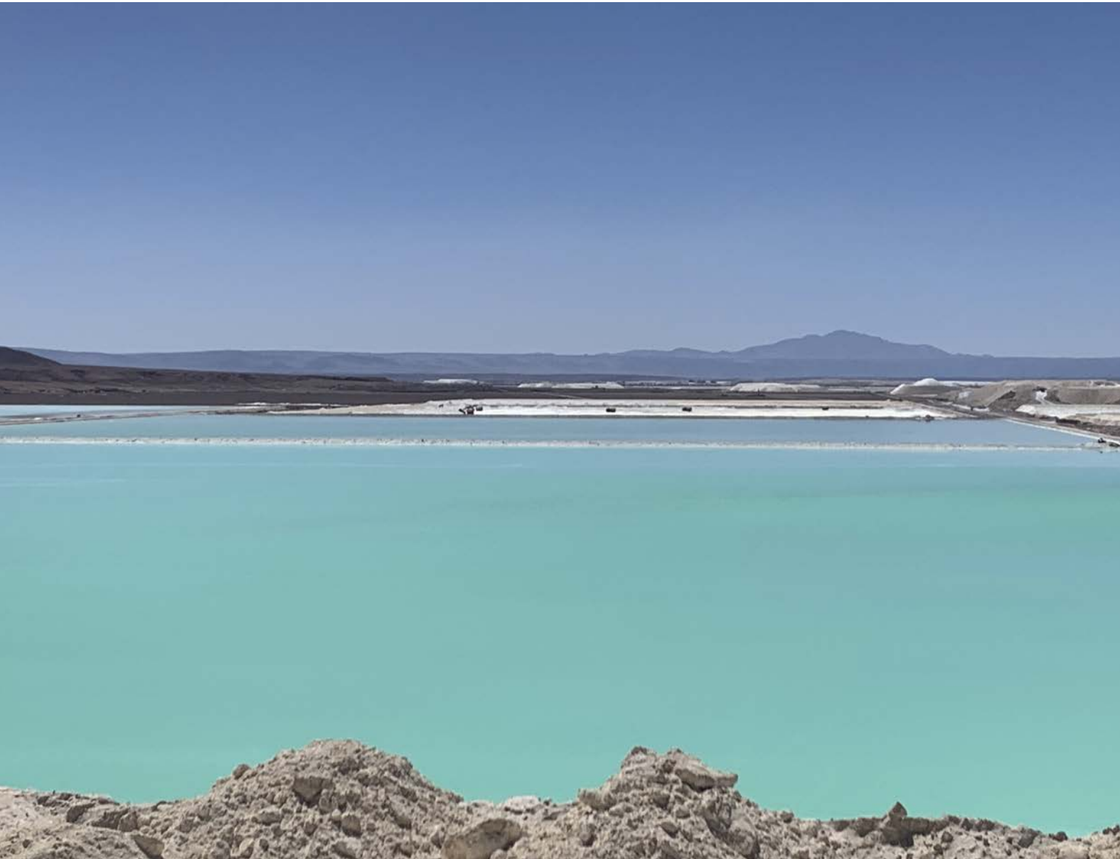
Evaporation ponds for lithium extraction from salt flats in Chile.
